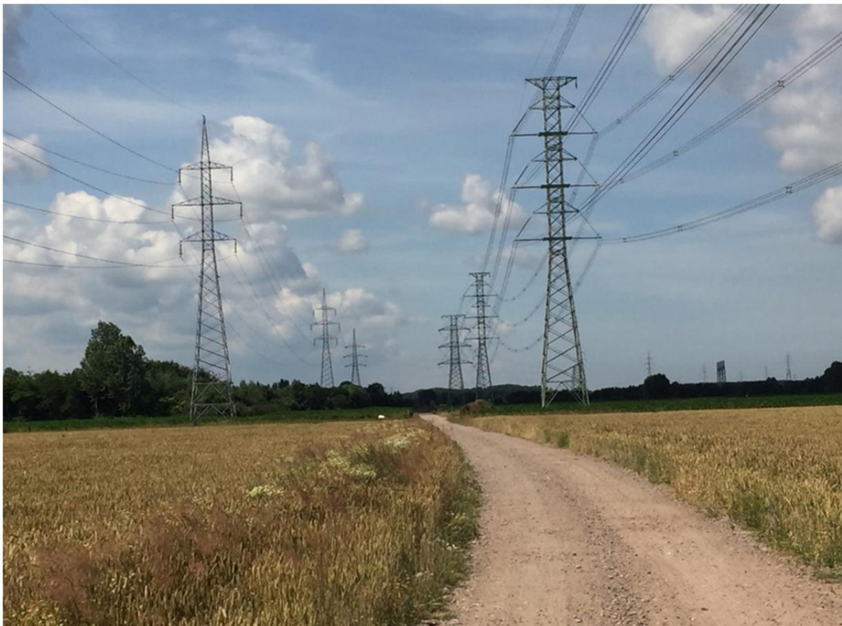
Figure: existing 150 kV line with new compact line 380 kV
