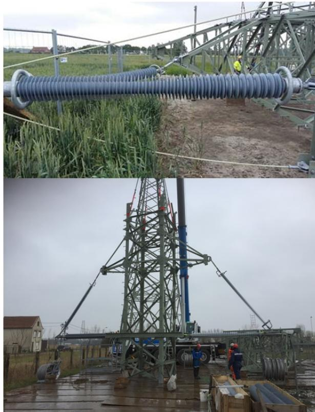
To avoid the pivoting of the cross-arms during pulling operations, a blocking system made of guy insulators without silicone has been developed and has proven to be efficient. Even if there are some risks to manipulate the unprotected guy insulators (gloves are requested), it was seen as a better inspection way to assess that there was no damage to the core and then it could do the job, what was impossible to be assessed when covered by silicone.
