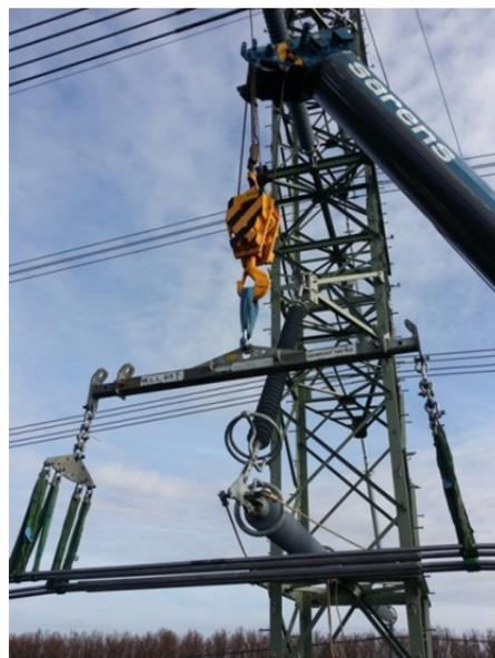
Normally it was not allowed to put a pulling machine just after a pivoting vee but only after a dead-end tower. Due to some difficulties on one location, it was required to test another working method which appeared to be satisfactory but not ideal by using a crane to limit the vertical force but mainly the longitudinal unbalance on the pivoting vee.
