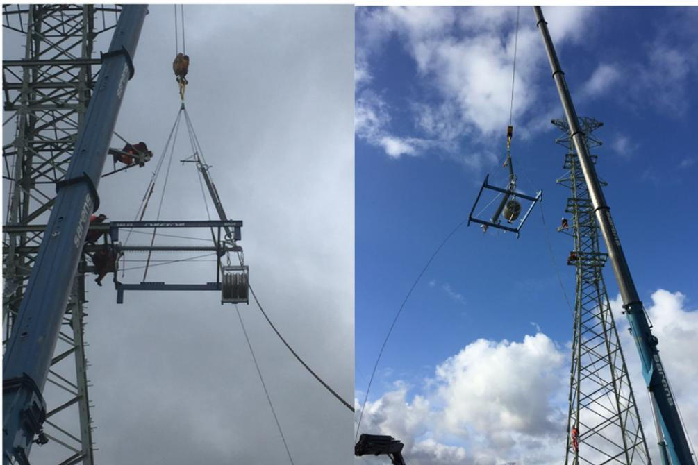
One contractor has developed a flexible mounting platform that fits for both pivoting and non-pivoting cross-arms of both suppliers. It is a very safe method that required some adaptations in the first stage but could lead to a quick installation of about 3 cross-arms per hour on an erected tower or one tower in half a day taking into account all the time requested to shift from one tower to the other one.
