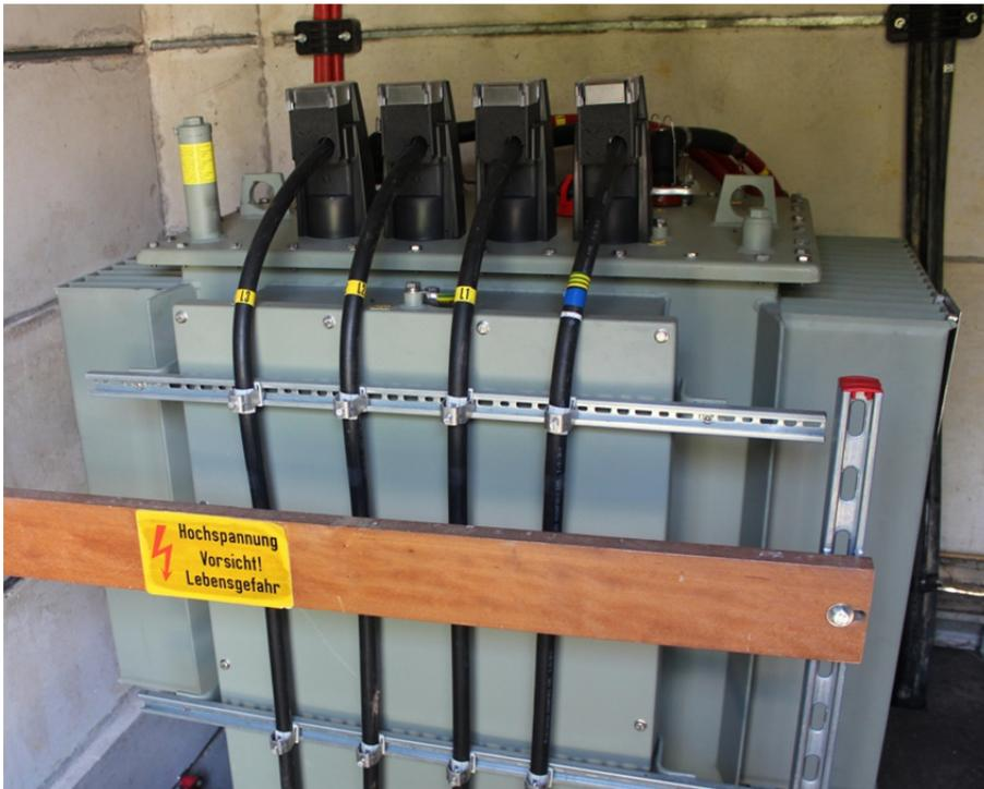
Picture 5: Regulated Distribution Transformer installation
