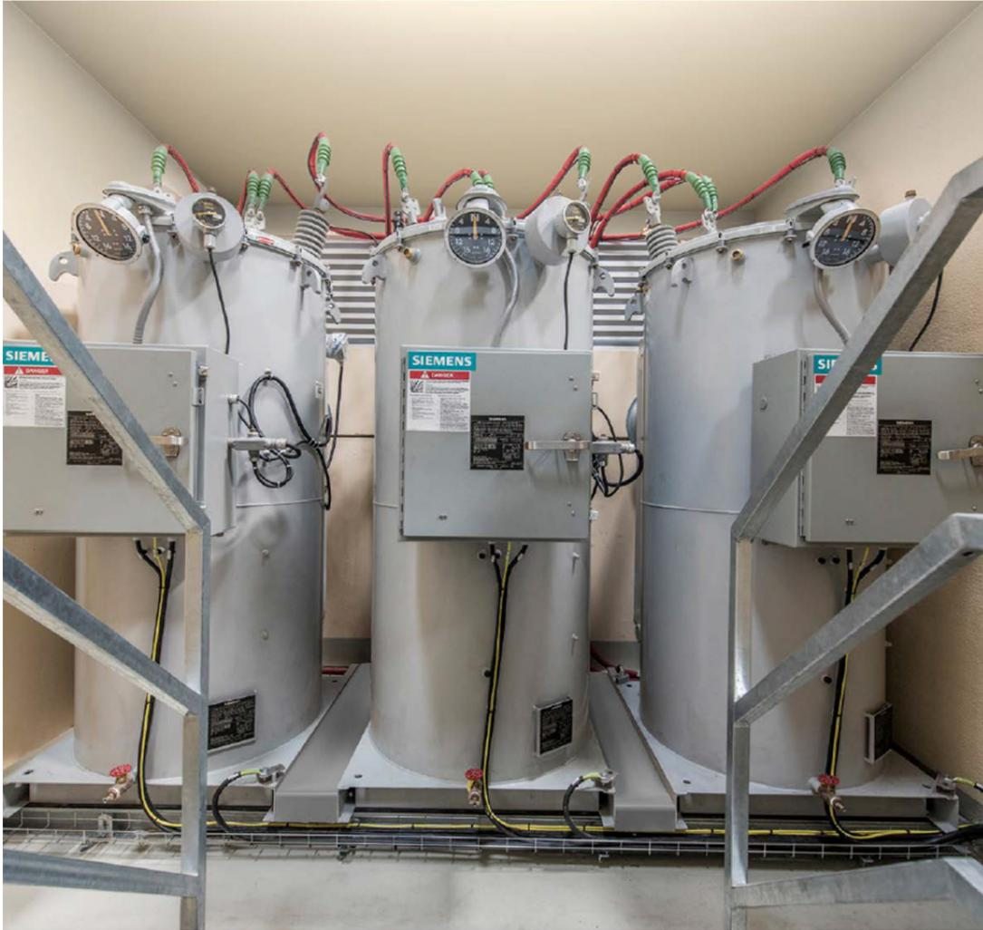
Picture 3: Line Voltage Regulator installation
