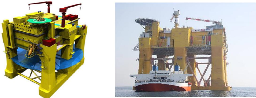
*Figure 11 A 3-D model (left) and photo (right) of the self-installing steel gravity base structure (GBS) platform for Dolwin2*
