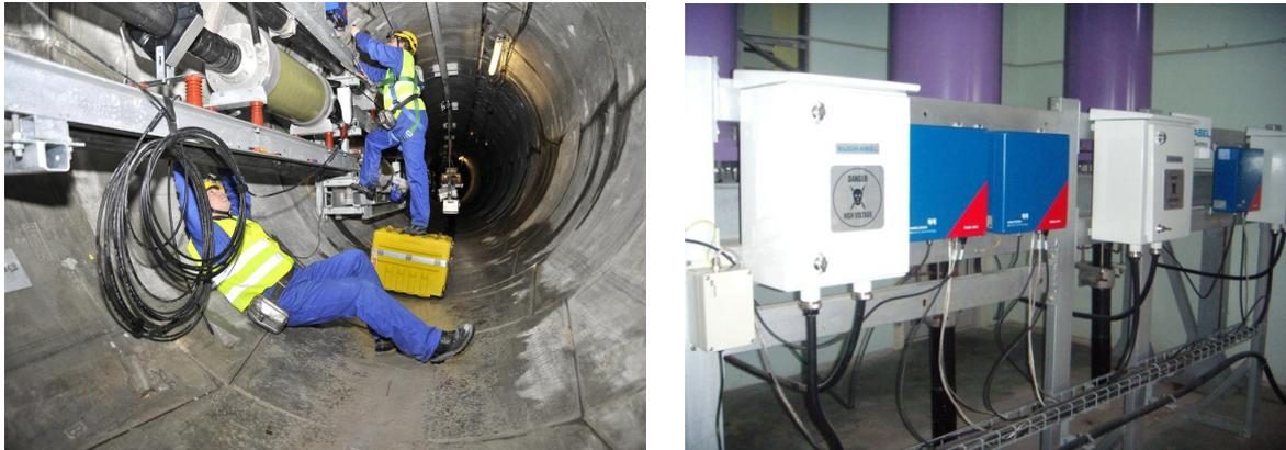
Figure 13: PD monitoring system installed in a cable tunnel or on 500 kV GIS XLPE cable terminations
