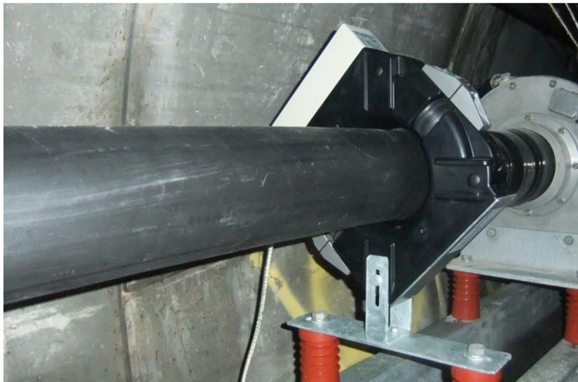
Figure 8: Inductive power supply at a 400 kV cable (single phase)
