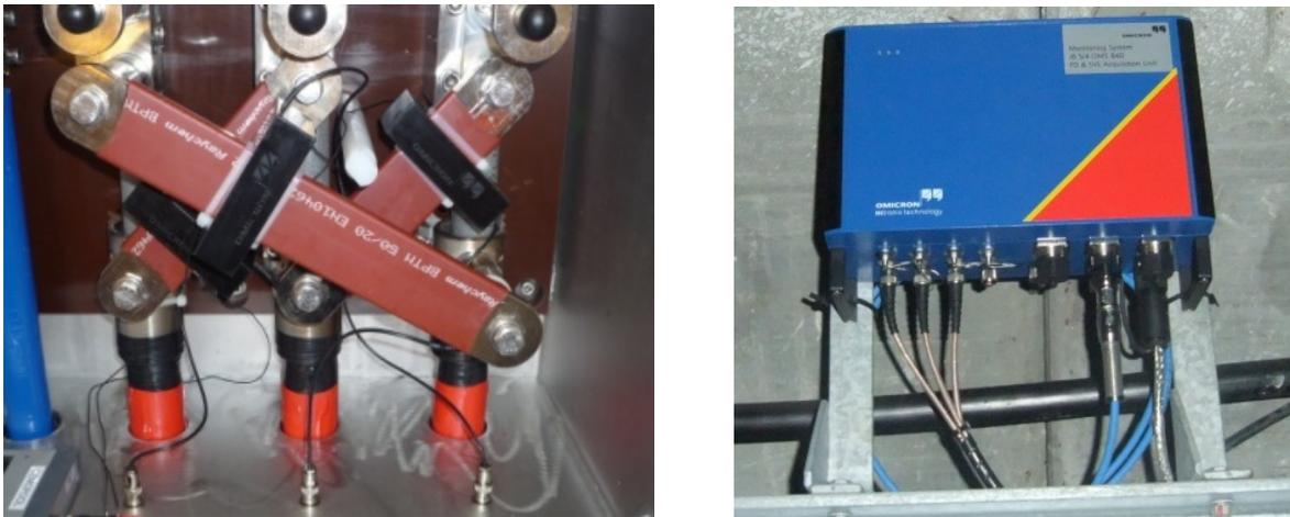
Figure 7: Example of HF-CT sensors in a XB-link (left) and one four channel synchronous PD acquisition unit (right)
