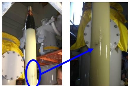
Tracking path as reason for partial discharges caused by foreign matter in the high voltage insulation system
