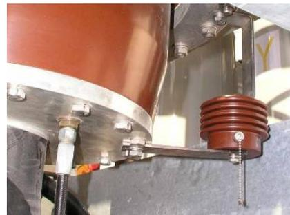
HV Termination with Decoupling Loop
