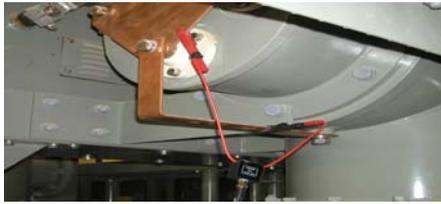
Fig. 1. UHF sensor adapted to a GIS grounding bar
