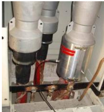
Fig. 15: On-site test set-up
