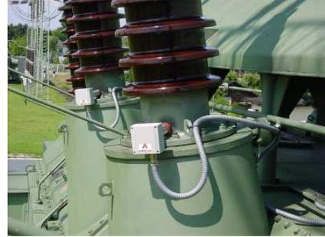
Fig. 4. Bushing voltage sensors installed on the measurement tap of the bushings
